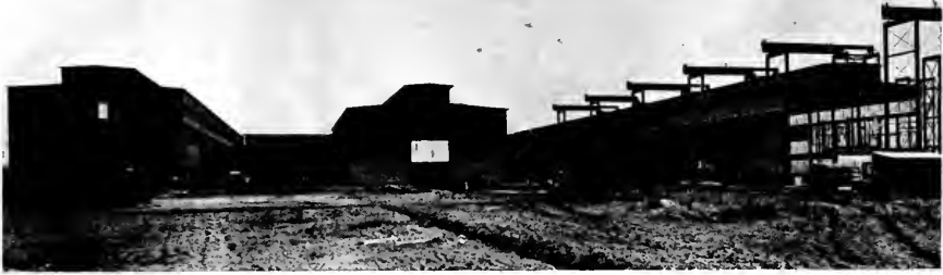
The large fabricating shop at the Sun Shipbuilding Company plant is built in the shape of the letter "H" and arranged for the continuous passage of raw material in one direction.
